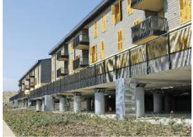
Fig. 22 Some completed buildings.
